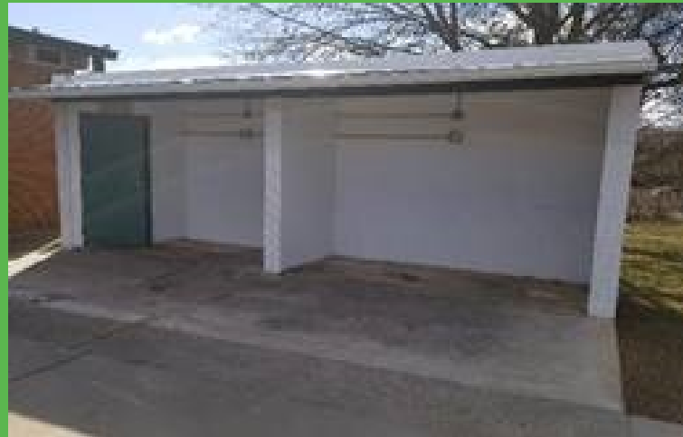
Pool Vending Hut Renovations
