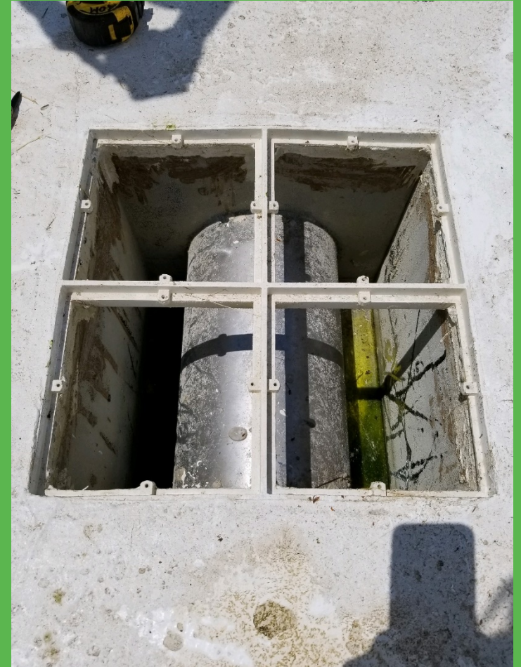
Drain Work in Main Pool
